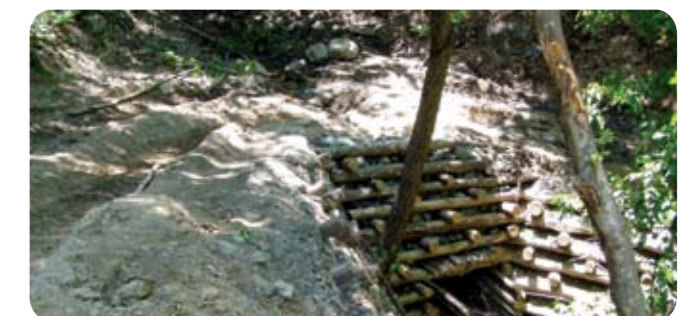
Waste wood fixes steep slopes in the mountain forests
